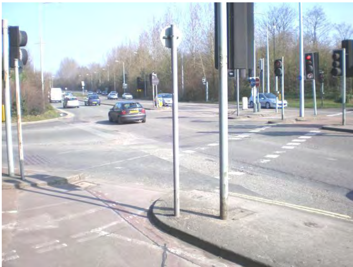
Figure 12.6: A35 Stoneham Way, looking north at junction with Wide Lane on the right
